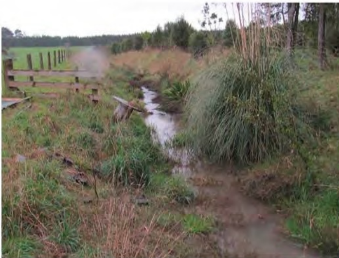
LOCATION D (FIG 2) - The existing northern stream channel will be enhanced to receive there – aligned north-eastern tributary
