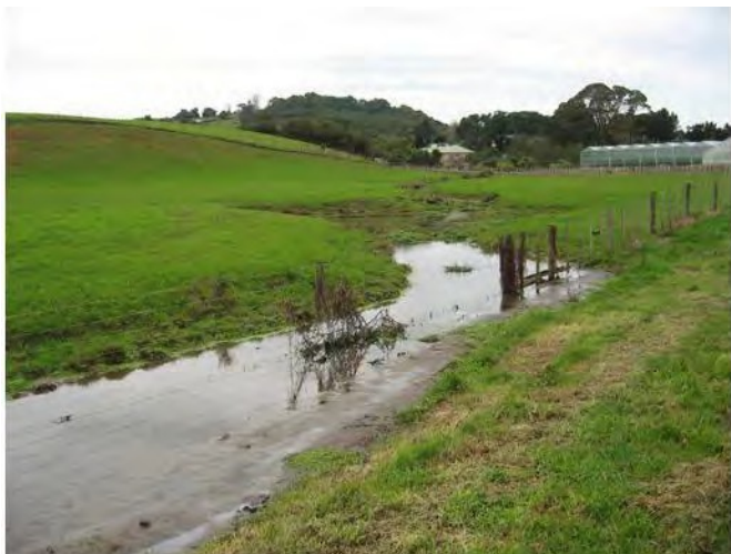
LOCATION F (FIG2)-The southeastern stream ponding behind a road culvert, 50 metres downstream of the proposed Willow Road Re-alignment
